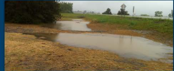
VTrans 75c I-89 Exit 19 N-Bound Off-Ramp
